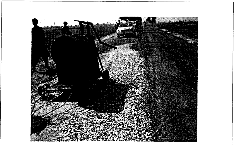
Photograph - 14 Repair work at the failed section is in progress (Aggregates are being spread to fill the depressions in the WBM layer, later TST will be carried out)
