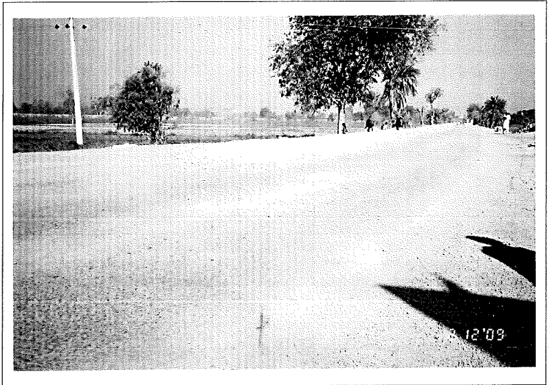
Photograph - 12 A newly repaired section of N-20
