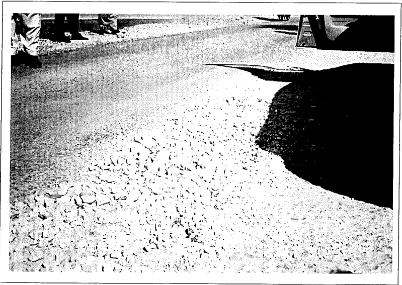
Photograph - 22 Repair work carried out with same size of aggregates for WBM layer.
